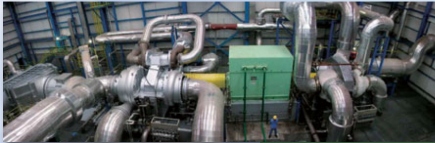
Air compressor (6-stage) and gas expander for P.T.A. plant
