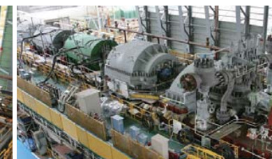
Mega Ethylene Plant
