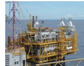
Offshore Gas Treatment Plant
